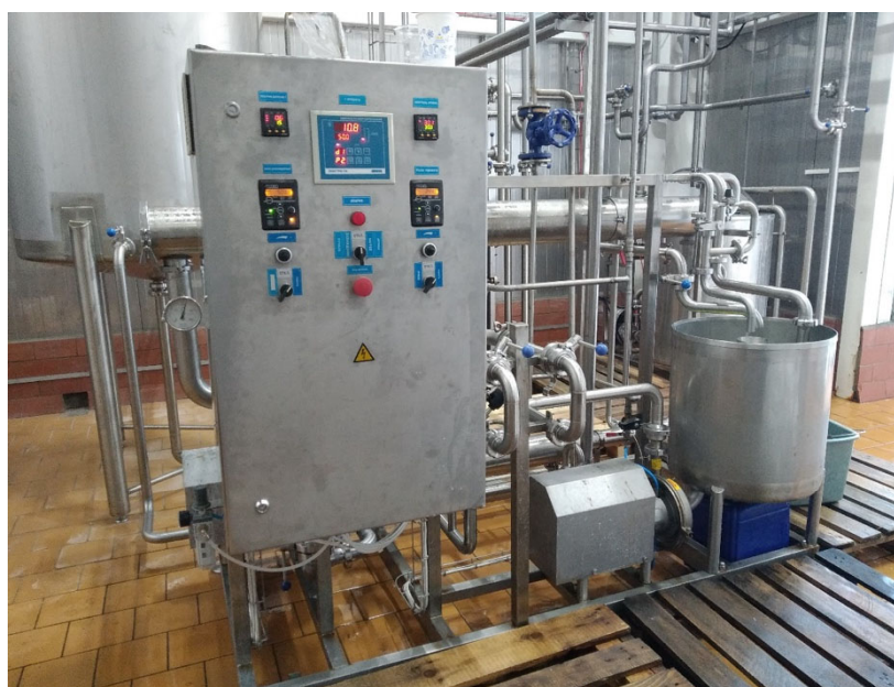
Fig. 2 Automated brine microfiltration unit type AUMF-1
